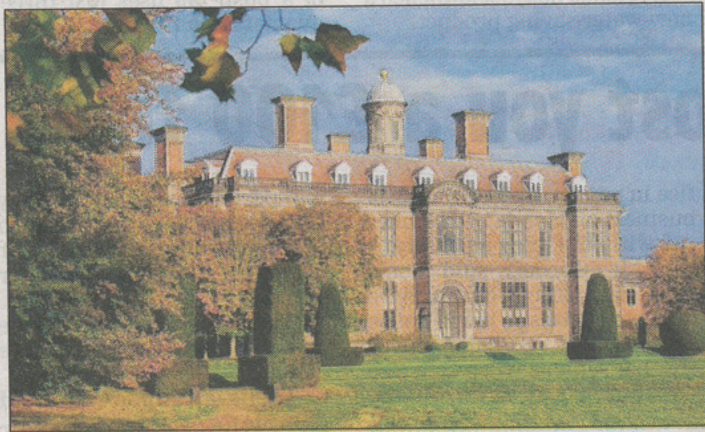
NEW-STYLE HEAT: Sudbury Hall now has bio-mass boilers.
